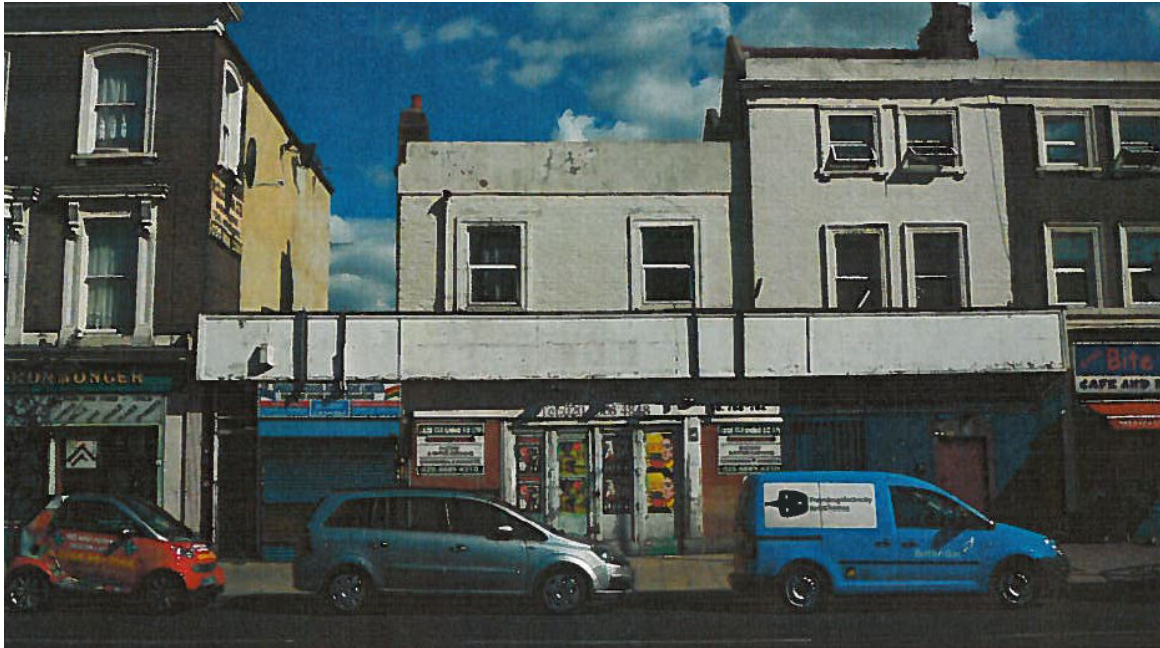
Existing Tottenham High Road Frontage
